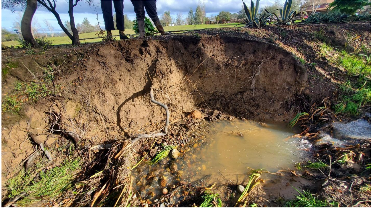
More stream bank erosion January 2023
