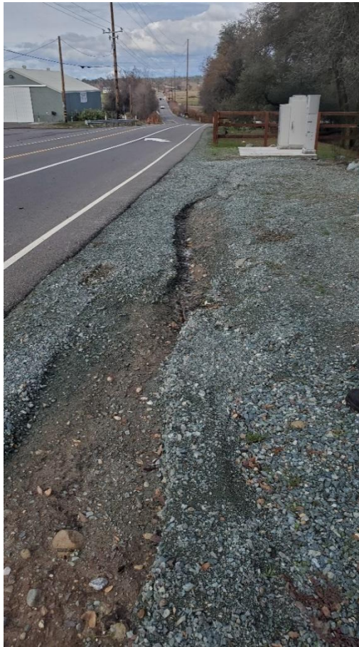
Erosion caused by stormwater runoff from storm in January 2023
